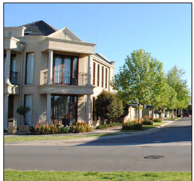
Where a footpath exists, an irrigation conduit is provided for you to link your home watering system to your front verge
