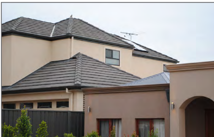
Ancillary structures should be located to reduce the visual impact from the street
