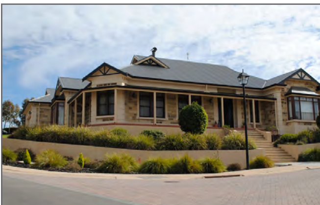
Use of lower terraced retaining walls is better than larger expensive walls
