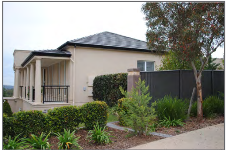
Colorbond fencing not to come forward of the main building line
